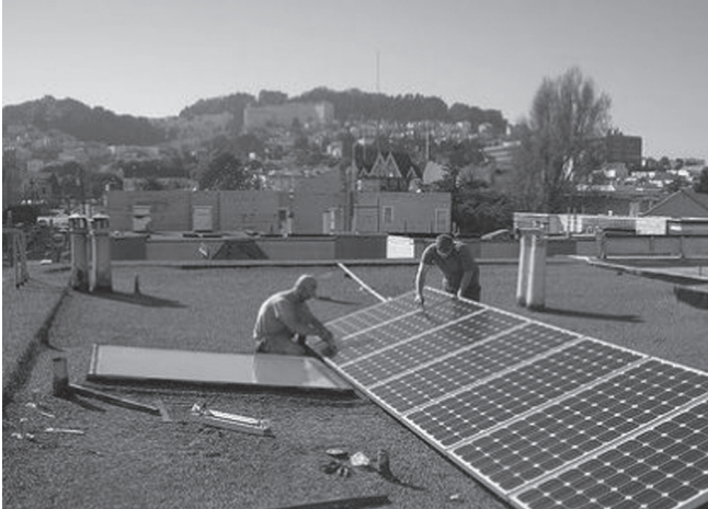
Workers constructing a rooftop solar installation. Photo courtesy of Stephhicks68.hubpages.com .
